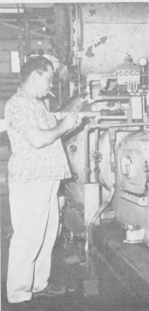
J. RASMIJN, controlman at the Compressed Air Plant, operates and services the compressors which compress 12,500 cubic foot of air per minute.
